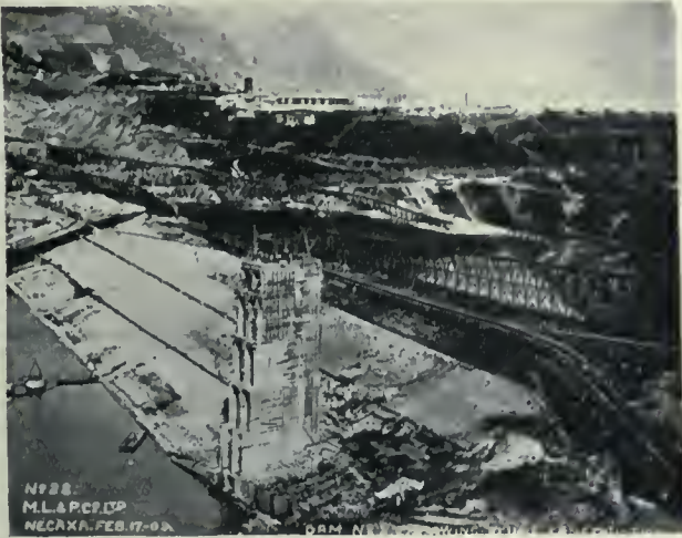
Necaxa dam from upstream toe showing sluicing trestles.
